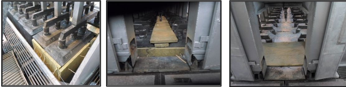
Figure 11. Insulation along long, short sides and centre.
