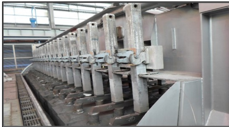
Figure 9. Anode alignment and anode placements.
